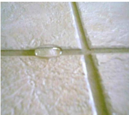
Above Left: Photo demonstrating water beading on sealed grout line Above Right: Photo showing partly sealed/unsealed Limestone
